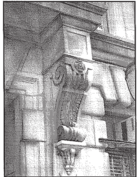
Figure 4: Below: a close up of the ornate carved stone bracket surrounding the entry on the east elevation of the building. (Photo: The Westerly Group, Inc. 2008)
