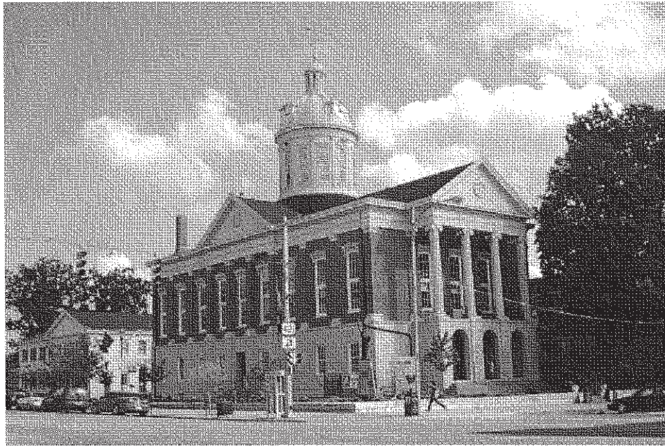
Figure 6. Jefferson County Courthouse, Madison, Indiana
