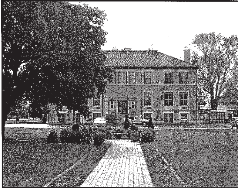
Photo of the East façade of the building (facing N. 4 th Street) The Westerly Group, Inc.2007
