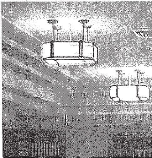
Fig. 7-16. Joining of remodeled to original ceiling molding at southwest corner of courtroom.
