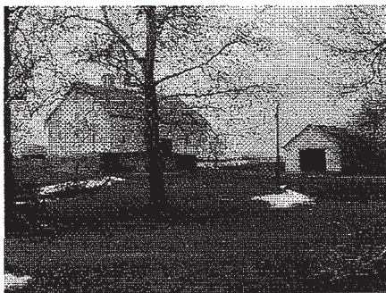
Figure 1d. Bank Barn from South
