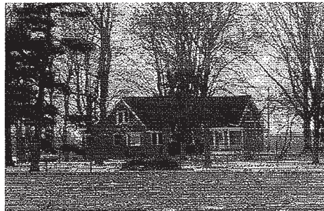
Fig. 5d. Garrison Home from the East.
