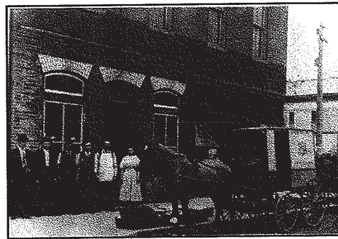
Fig. 27 Burch Grocery, c1909. The west storefront (Bass Drugstore) has been remodeled with cast iron columns. Source: Grocery Stores file, Mooresville Public Library.
